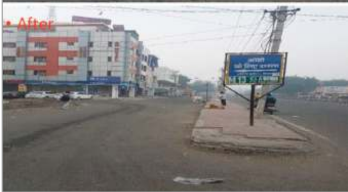
Road repair works conducted by Honda to reduce accidents
