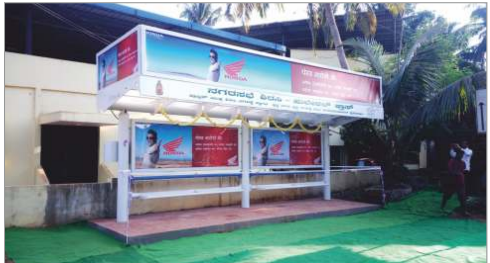
Bus Shelter at Karnataka
